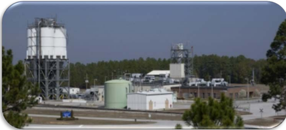
Fig. 4. View of the Saltstone Facility
