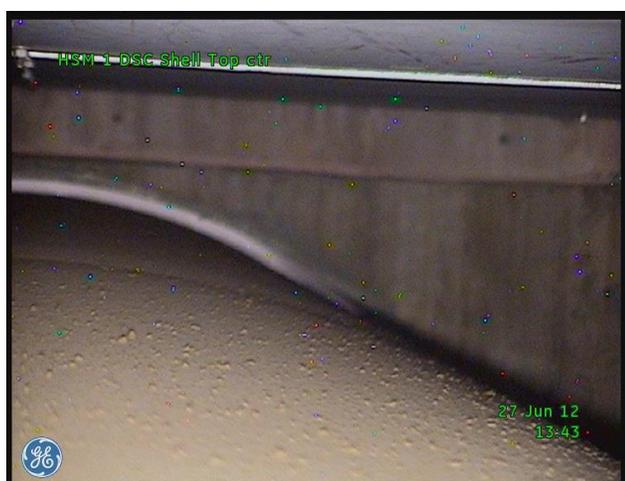
Figure 3. Dust on top of canister at Calvert Cliffs
