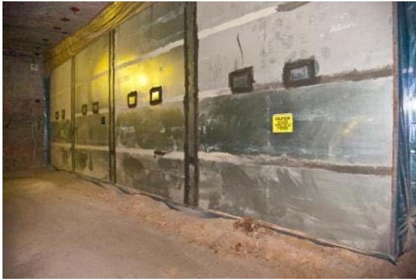
Figure 5. Steel bulkhead doors in routine use in the Waste Isolation Pilot Plant underground facility.
